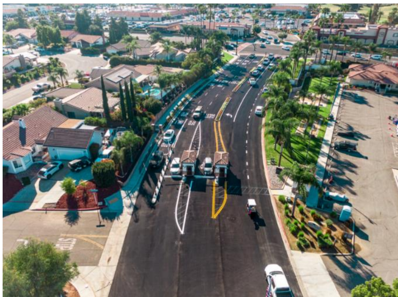
MAIN GATE REPAVEMENT
